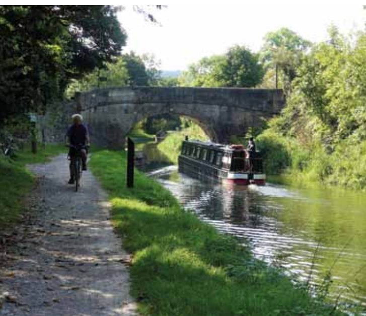
Cyclists, Boat & Bridge
