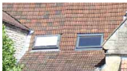
Modern rooflights can detract from the historic character of buildings
