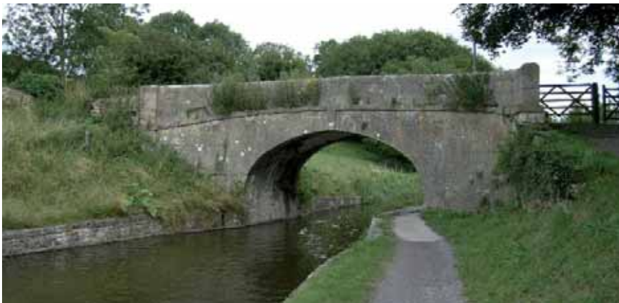
The canal and associated structures contribute to the attractive rural setting of the Conservation Area
