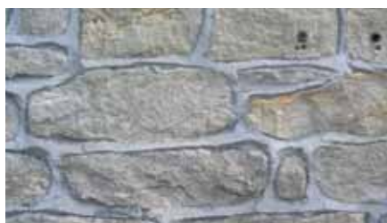
Neglect of boundary walls, cement mortar repairs or unsuitable pointing can detract from the character of natural stone walls
