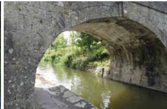
Ferry Lane Bridge
