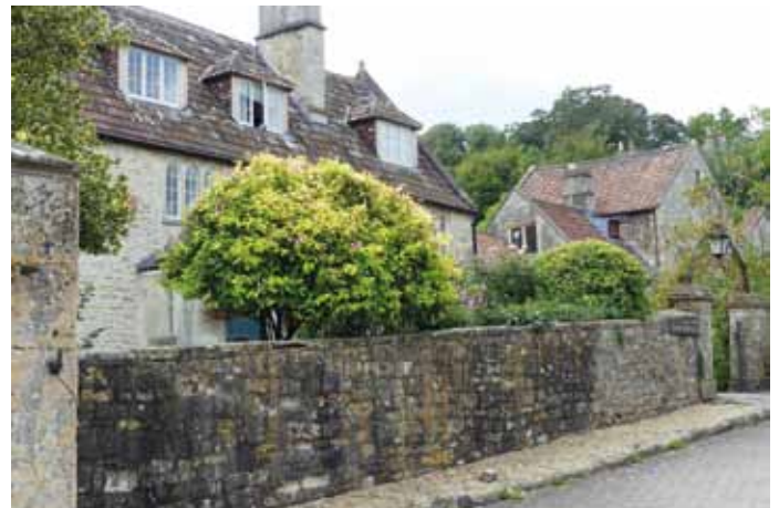
Manor Farm House and the Dovecote
