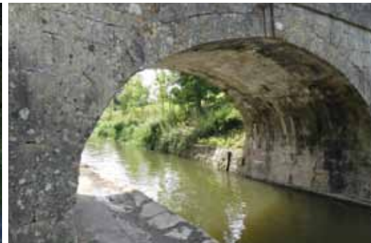
Ferry Lane Bridge
