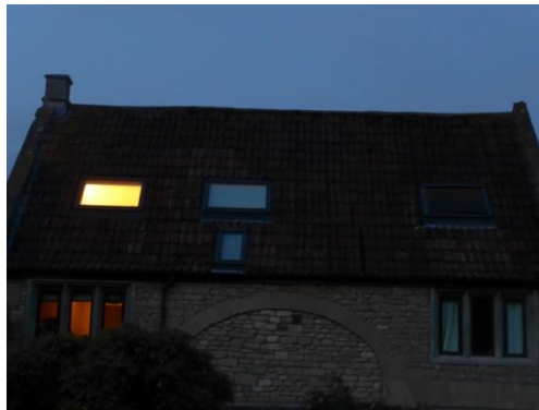
Left to right : (1) no blind; (2) internal venetian blind; (3) internal and external blind
